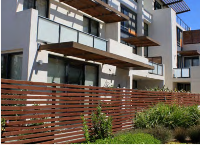
Figure 3F.9 Fencing of ground floor apartments should not be solid to allow for surveillance of common open space and the public domain
