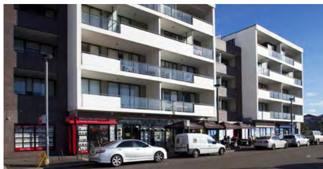
Figure 3J.1 This development provides green open space on top of the car park structure (top photo). The ground level facing the street is 'wrapped' with retail and commercial uses (bottom photo)
