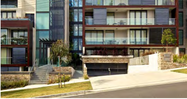
Figure 3H.3 Vehicle and pedestrian access should be clearly separated to improve pedestrian safety and comfort
