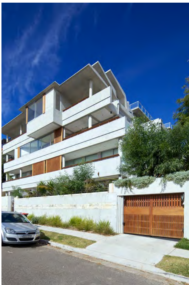
Figure 3J.15 The impact of car parking and vehicular access points on the streetscape should be minimised
