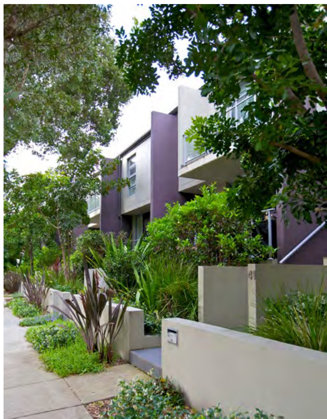
Figure 3C.3 Planting can be used to soften the edges of raised terraces to the street
