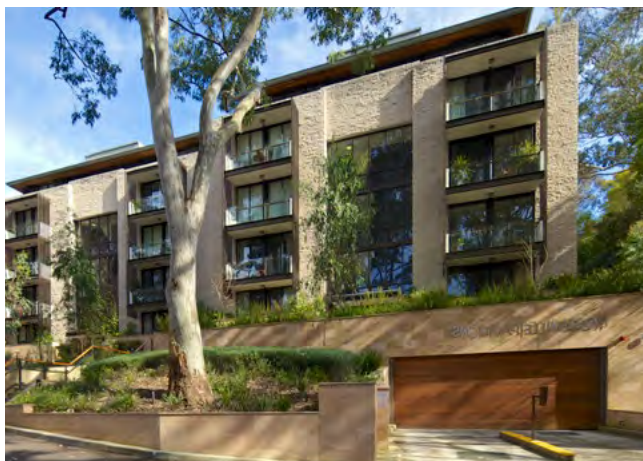
Figure 4H.4 Bedrooms should be located at least 3m away from noise sources such as driveways and garage doors
