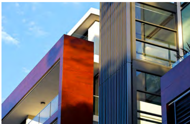
Figure 4M.3 Building articulation such as balconies and deeper window reveals provide visual interest to the facade
