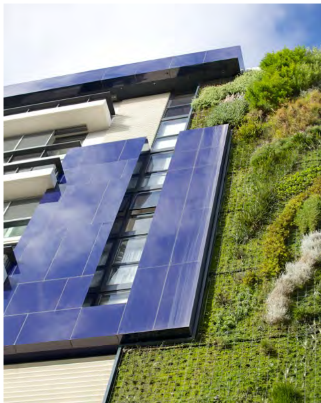
Figure 4P.1 Green walls and facades make positive contributions to the environment and to urban amenity more generally. They can also improve the sustainability performance of a building
