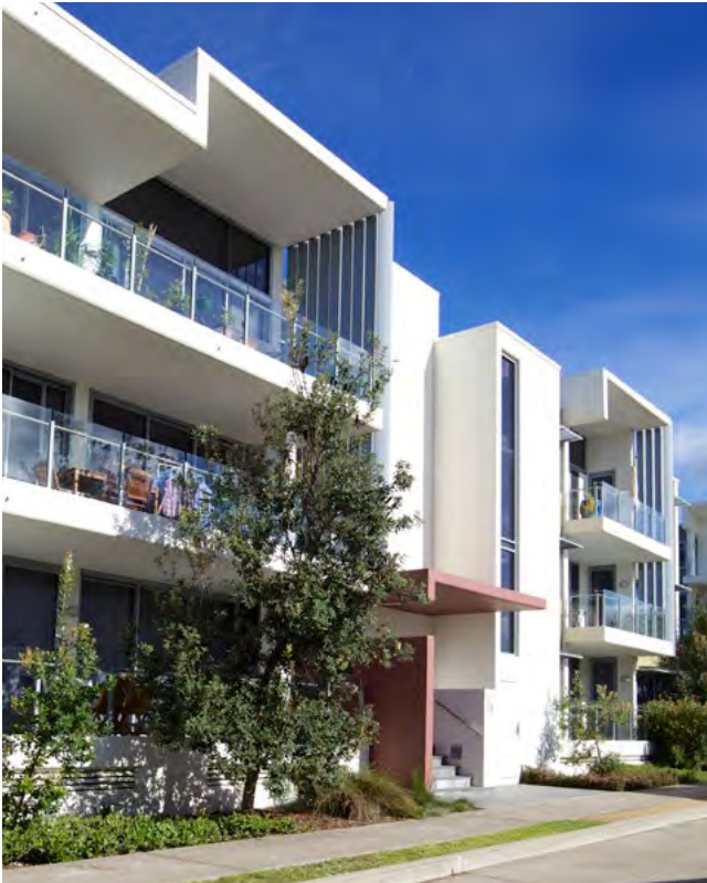
Figure 4C.4 Differing ceiling heights are an opportunity to provide visual interest in the building facade
