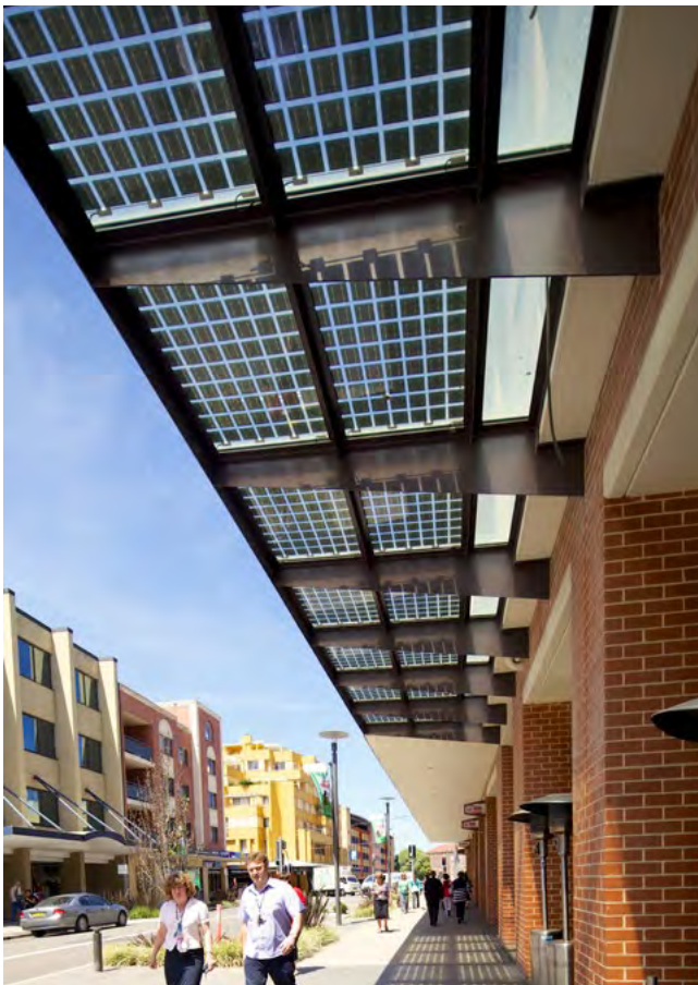
Figure 4U.5 Environmental technology, integrated into the overall design, adds to the sustainable performance of buildings
