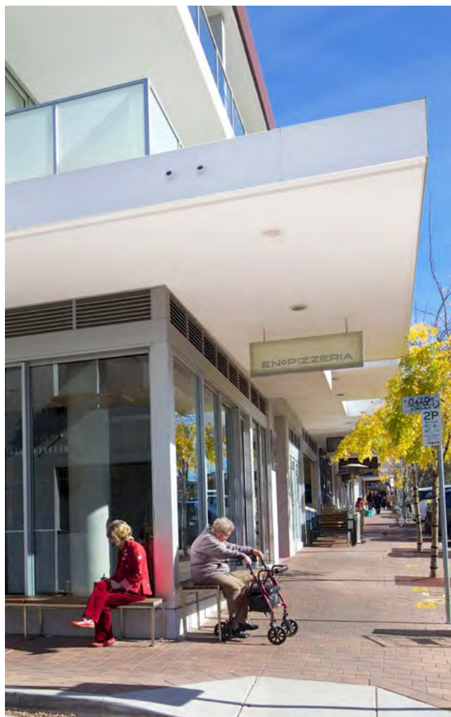
Figure 4T.2 Awnings should be designed as an integral element of the building and incorporate lighting for added safety
