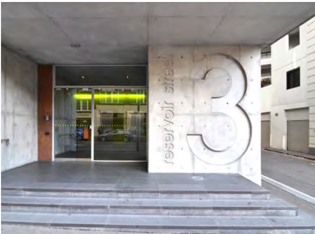
Figure 4T.4 Building address signage can be integrated as a feature of the facade design
