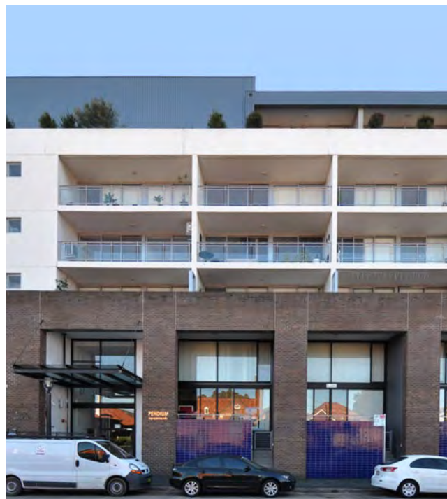
Figure 4X.1 Building facades should use materials that are long lasting and weather well over time, such as brickwork, tiles and glass
