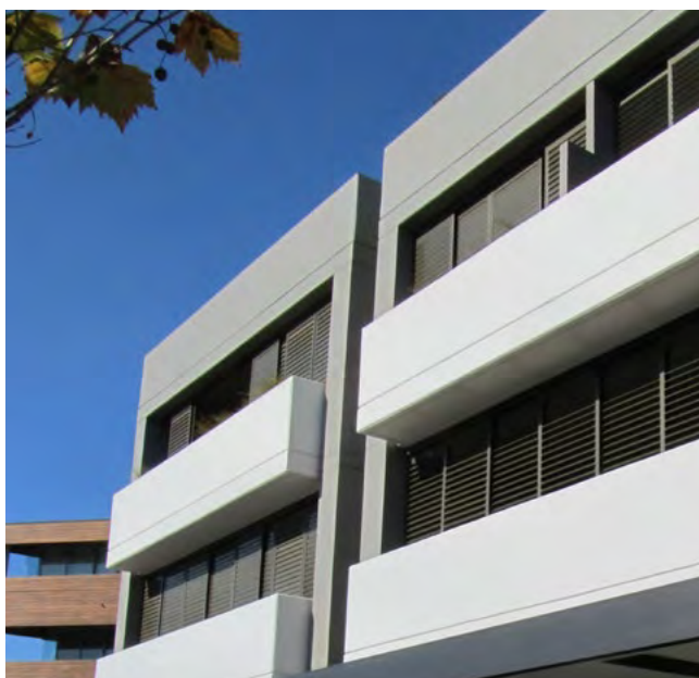
Figure 4B.2 Operable balcony screens allow occupants to customise their environment and regulate access of natural light and ventilation
