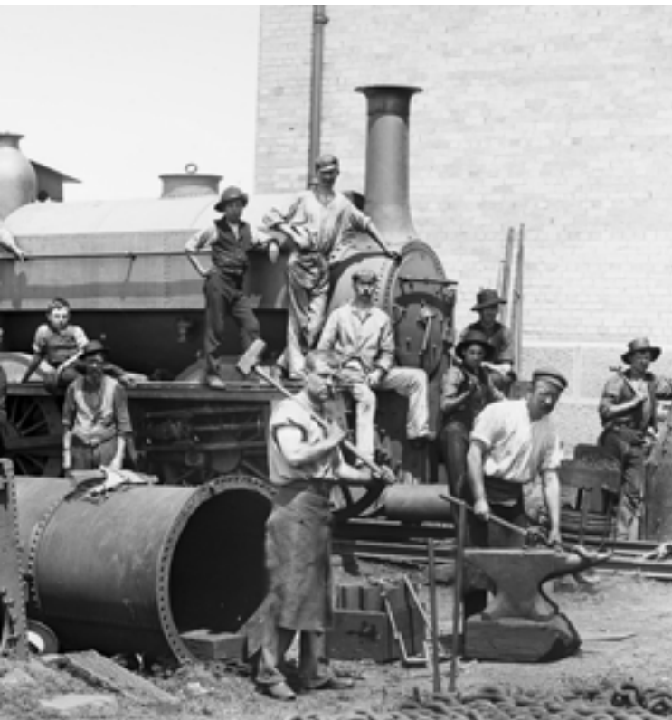
Locomotive engine being repaired outside the Hydraulic Engine House, Carrington, courtesy of the Snowball Collection
