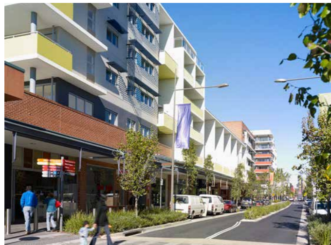
Figure 26: Proposed location of mixed use retail & residential, and desired character and built form
