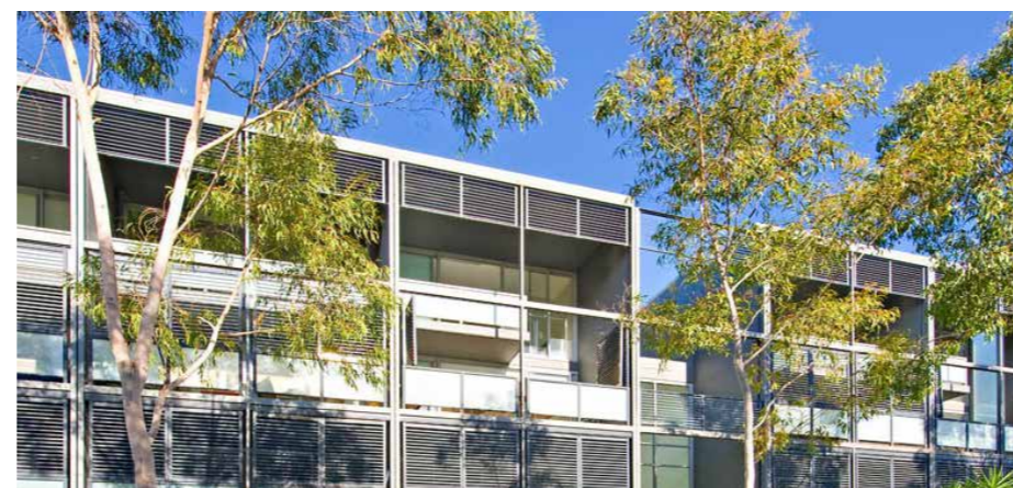
Figure 24: Proposed location of medium rise residential, and desired character and built form
