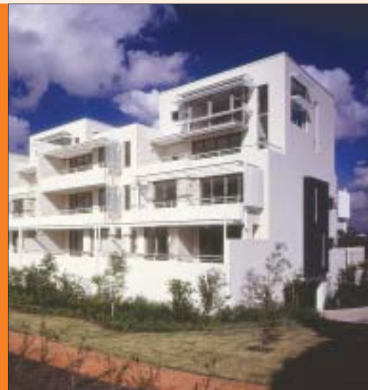
03.38. Sun shading is an integral component of the building form and facade design.
