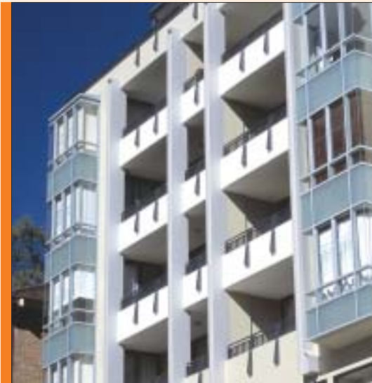
03.12. Primary balconies provide generous shaded outdoor living areas and add depth to the facade.
