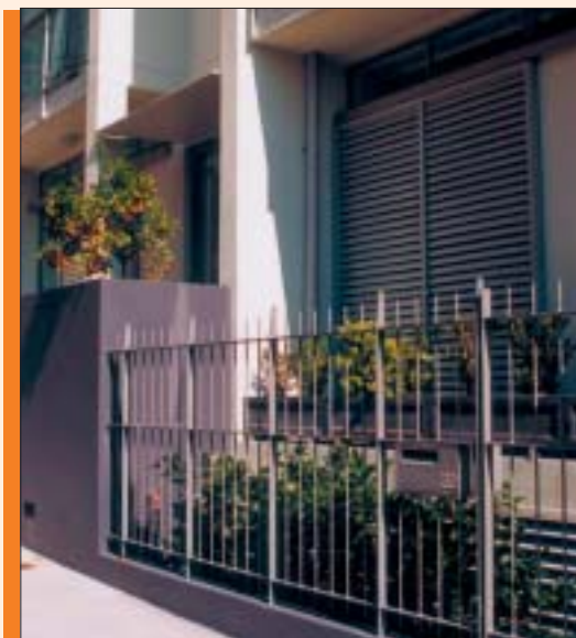
03.23. Street level metal picket fencing with planting provides screening to car park ventilation louvres.
