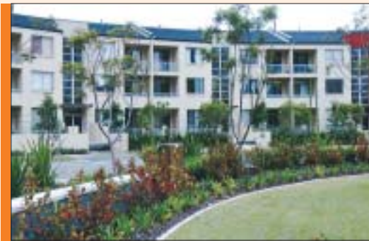
03.28. The use of multiple lift and stair cores promotes more entries along a street and articulates a long building facade.
