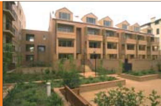
03.48. The more traditional design of this elevation uses a variety of repeated forms and a restrained material palette.
