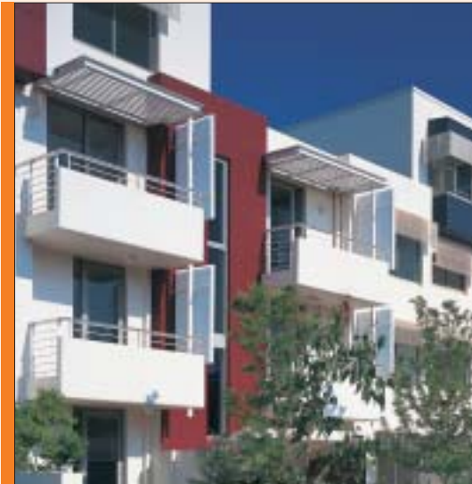
03.13. The detail design of these partially solid balustrades, sun shades and privacy screens contribute to the overall facade composition.
