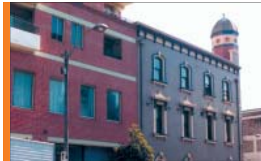
A4.14. A consistent parapet height and similarly proportioned windows enhance the relationship between the new and the old.
