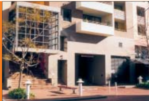
02.53. This elevation treats the carpark entry as part of the whole elevation. It narrows the width of the entry and defines an opening in proportion to the other facade elements.
