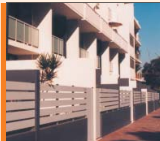
02.48. Multiple private entries along a street activate the street and create visual interest.
