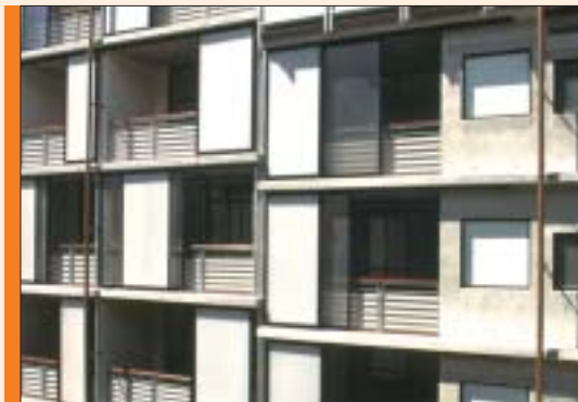
03.14. The operable screens increase the usefulness of these balconies by providing weather protection, daylight control and privacy screening.
