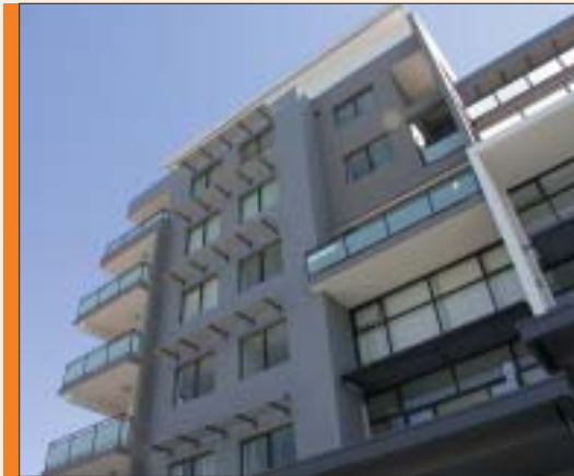
03.50. Use of varying facade alignments and sunscreens articulate the taller mass of this building.
