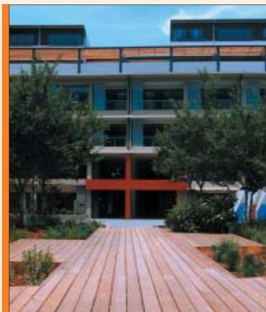
02.45. This well-defined entry is differentiated by a change in colour from the surrounding facade.
