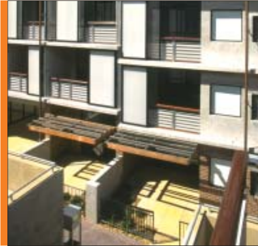
02.43. Building elements provide privacy between spaces - pergolas limit overlooking, and solid walls and sliding screens limit horizontal views.
