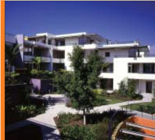
02.18. The site's topography has been used to create a series of smaller more intimate spaces using retaining walls and planter beds, which step down across the site.
