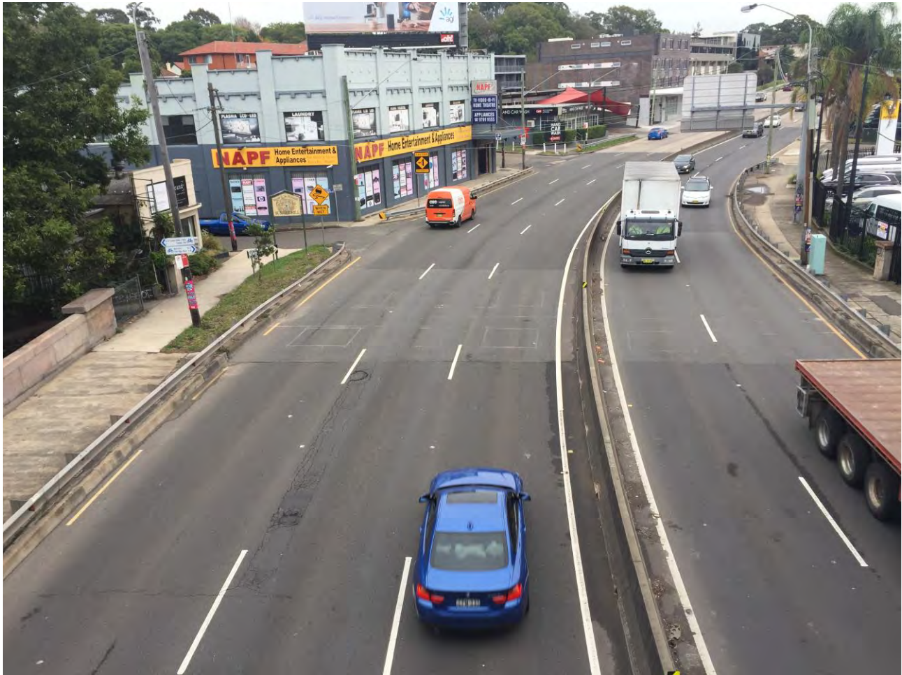
Figure 12-13 Parramatta Road at Taverners Hill
