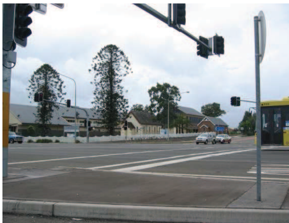
Windsor and Rouse Roads Intersection
