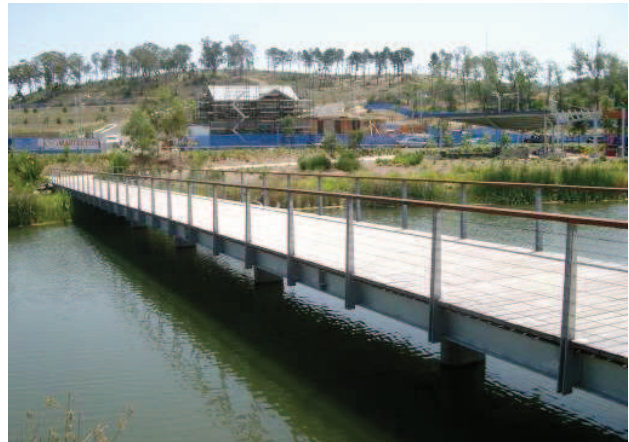
Boardwalk at Nelsons Ridge
