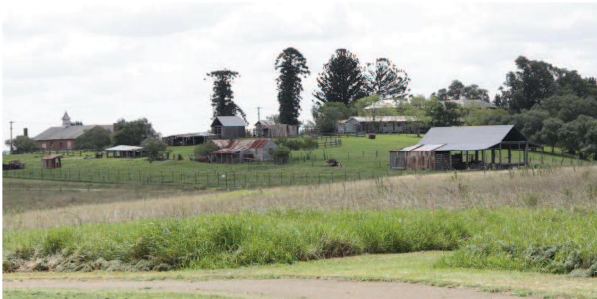
Outbuildings within the Estate
