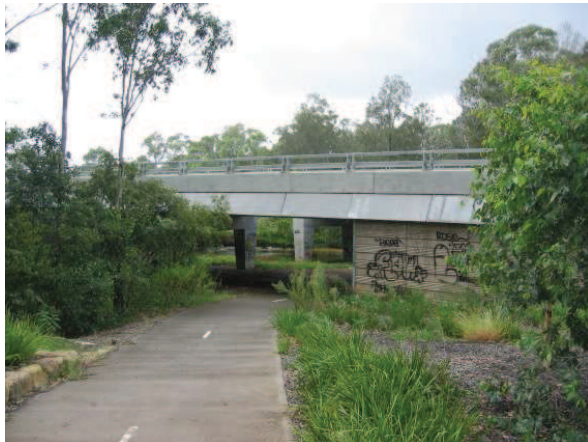
Pedestrian and Cycleway under Windsor Road
