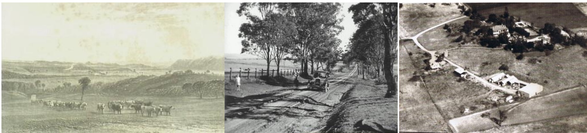
Figure 3.2 Left to right: 1840 sketch depicting the Cowpastures. (Source: Camden History by John Wrigley); 1928 view of Cobbitty Road. (Source: Camden Local Studies Library); and the internal roads of the Oran Park Estate in 1972. (Source: Camden local Studies Library)
