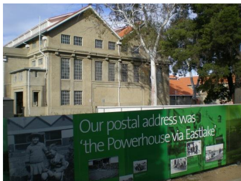
Site hoarding with interpretation messages during construction, Canberra Glassworks.
