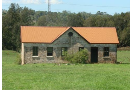
The coach house, a robust adaptive re-use opportunity for in community/commercial use
