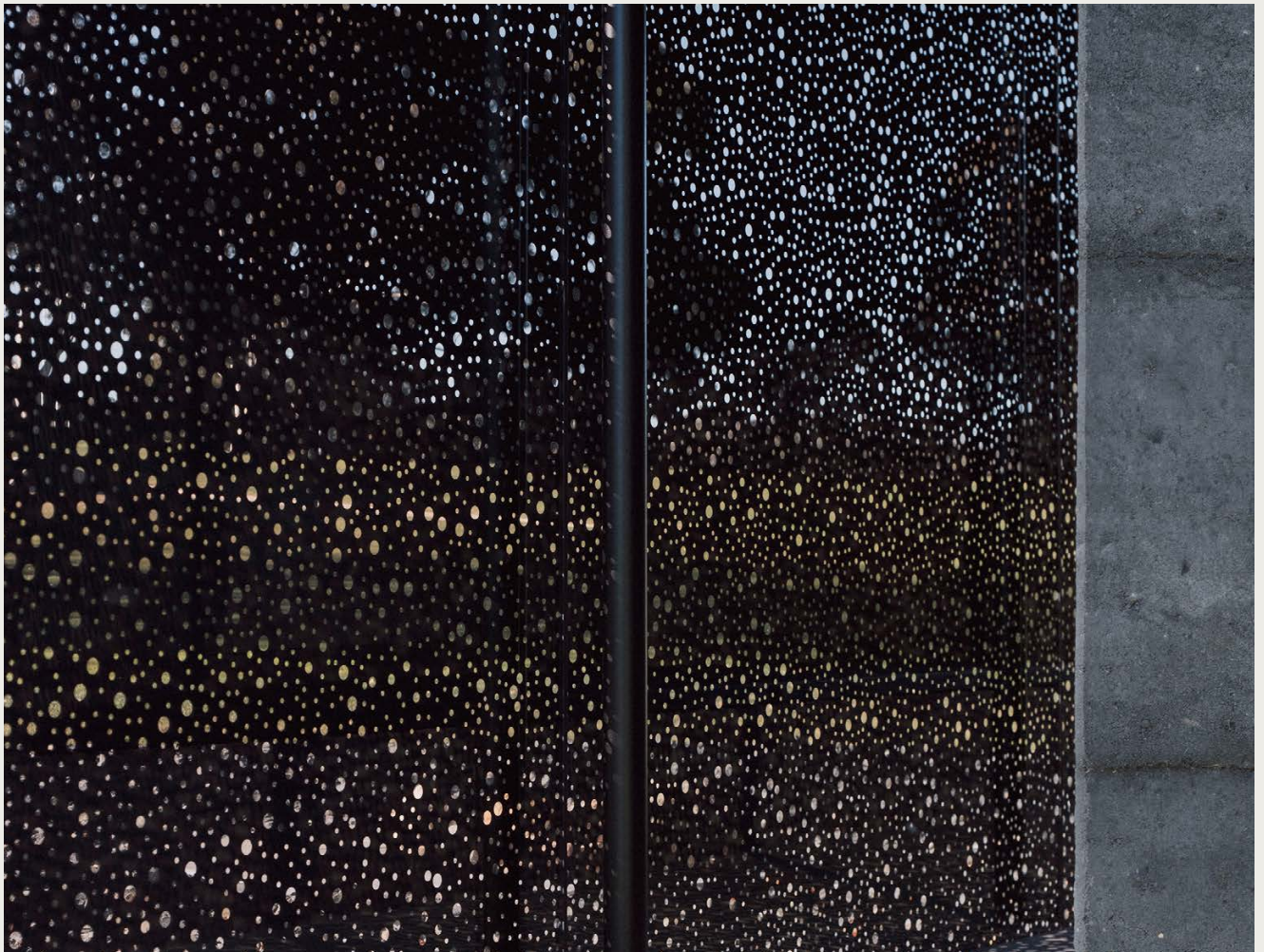
A 2-way mirror glass 'veil' filters eastern morning light into the pavilion. Image: Ben Hosking.
