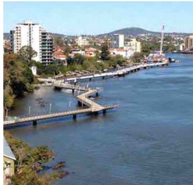
Light weight structures on Brisbane Riverwalk create a continuous and unique water’s edge for pedestrians and cyclists.
