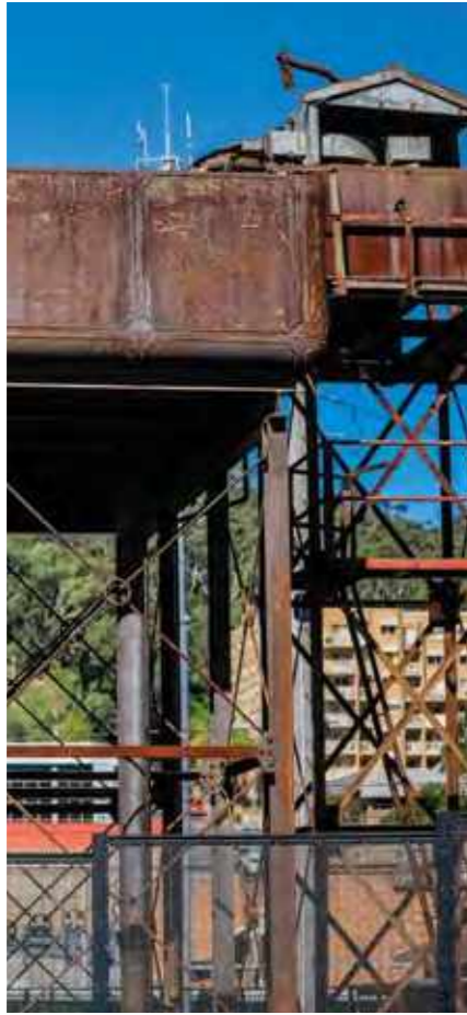
1. Rail character maintained.
