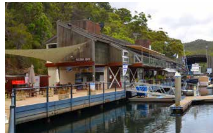
Akuna Bay marina building
