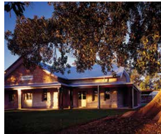
Wilcannia Health Service successfully provides a new health accommodation facility within an existing building. Image: Brett Boardman.
