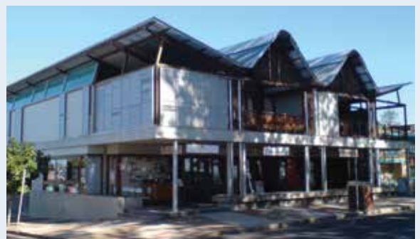
The design of a commercial infill site on Bay Street, Byron Bay responds to the warm subtropical climate of the region and contributes to the area’s local character. Borrowing elements from regional vernacular buildings, the project combines verandahs, slatted screens, and corrugated iron roofs to create generous and flexible outdoor rooms that can be used by owners, tenants, and customers in all weather conditions. Image: Troppo Architects.
