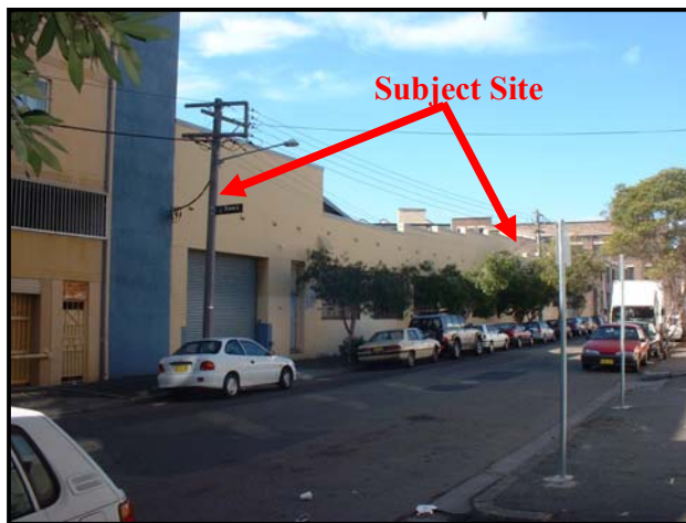
Hudson Street - view east of the existing building.
