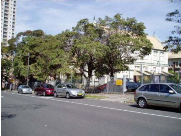
Photo 1: Site viewed from George St looking south west (shows Building B)
