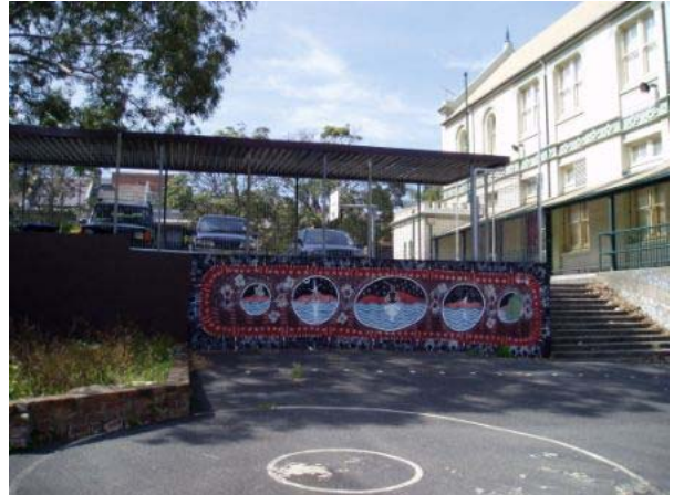
Photo 8: Building B and awning looking east.
