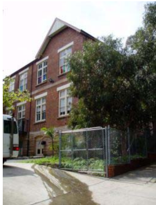
Photo 12: Western elevation of Building A looking north east
