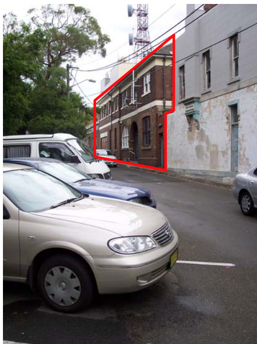
TURNER ST - VIEW FROM EAST - POLICE STATION
