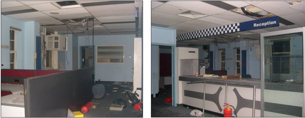
Figure 6: Interior views of the Police Station
