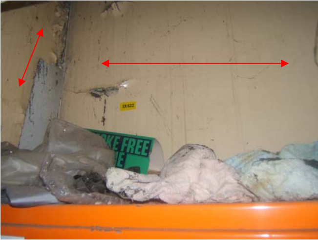
Photograph 18: Internal paint work to walls within electrical cupboard.
