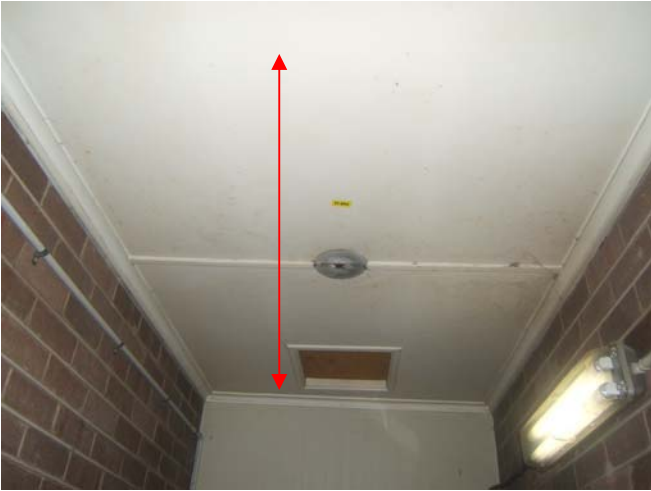
Photograph 14: Fibre Cement Sheet wall lining within Electrical cupboard.
