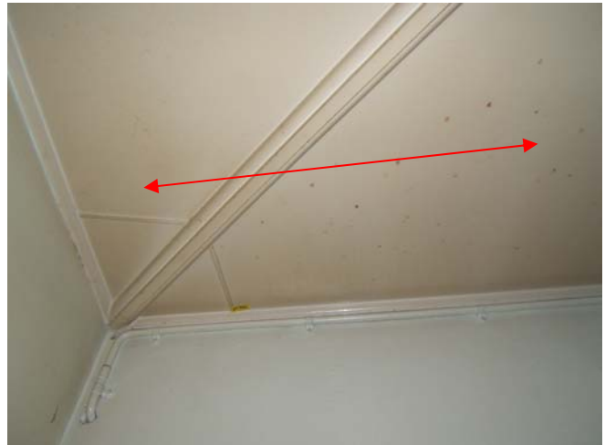
Photograph 6: Waterproof membrane on east side only of ground floor within ceiling space.
