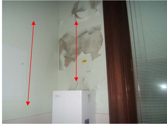
Photograph 19: Internal paint work to walls in DV room.
