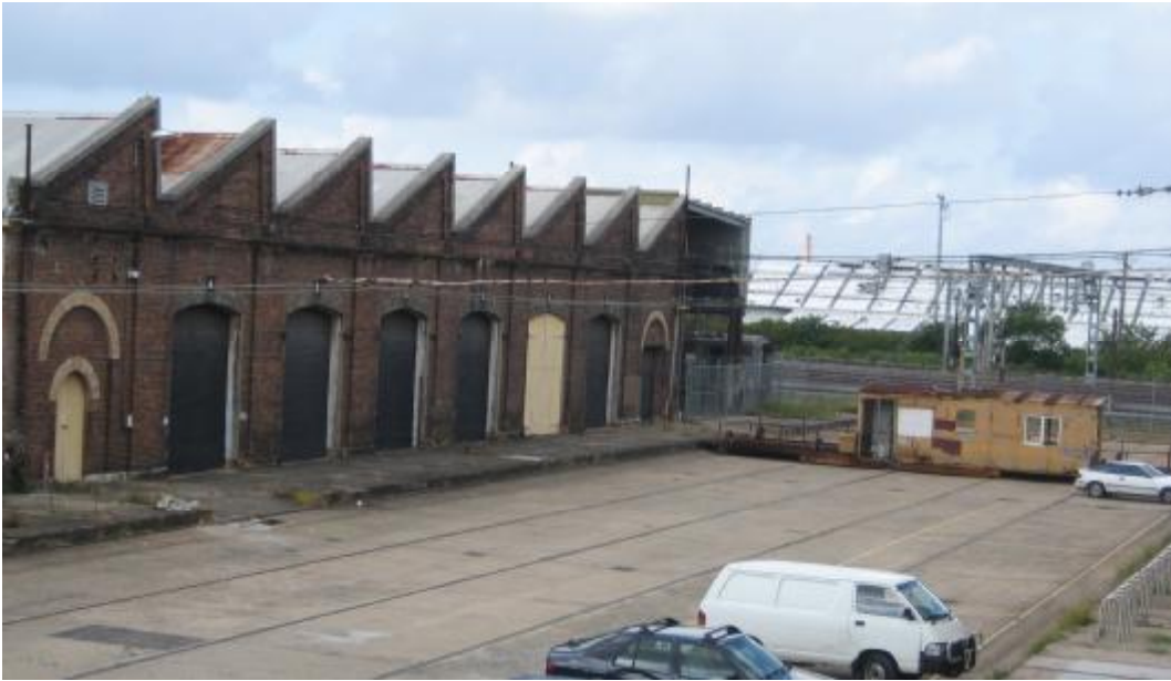
View looking south towards the rail corridor and ATP. Traverser 1 in foreground and Paint Shop in background.
