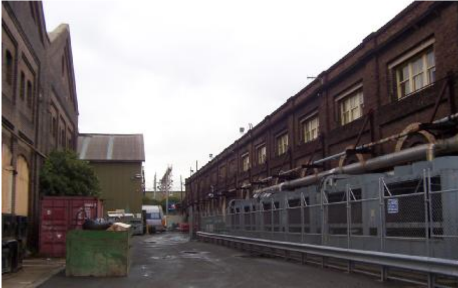
Corridor between Locomotive Workshop (right) and XPLOER Endeavour Service Centre (left background).
