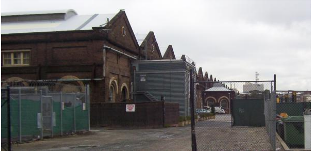
South western corner of the Locomotive Workshop and general area where bridge may land.
