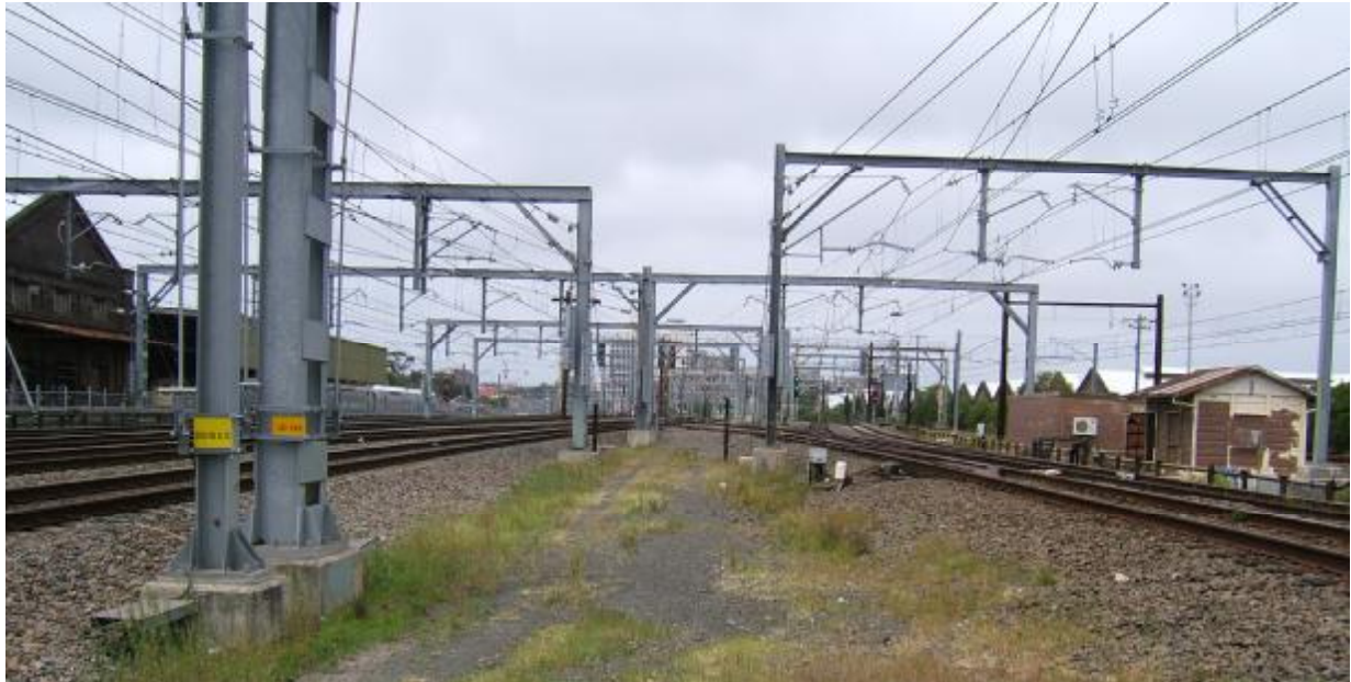
View along railway corridor looking east. ATP on the right and North Eveleigh on the left.
