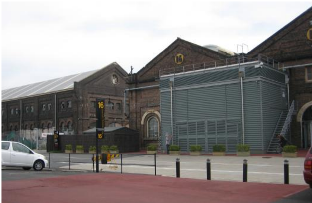
Locomotive Street and future location of proposed open space in foreground and Locomotive Workshop (right) and Large Erecting Shop (left) in background.
