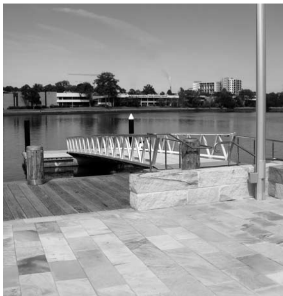
New public pontoon along Parramatta River at Meadowbank
