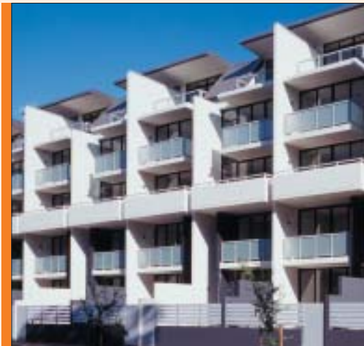
02.44. Lower level balconies have solid balustrades, limiting views from the street. Higher level balconies are set back beyond pedestrian sightlines and therefore glazed balustrades are appropriate.
