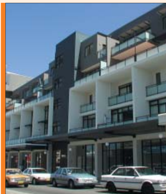
02.46. The facade of this building distinguishes the residential entry from the commercial shop fronts with a vertical element.
