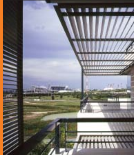
03.37. A combination of louvres provide shading for different times of the day.
