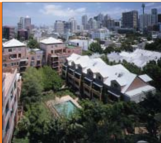
03.54. A variety of roof forms, pitched roofs with dormers and towers are used to reflect roof forms of the surrounding urban context. Service plantrooms are well concealed.
