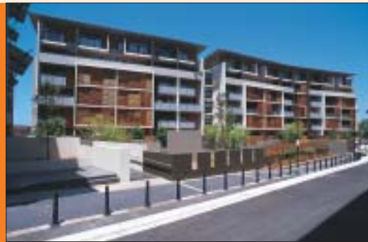
03.47. This facade balances strong horizontal and vertical framing elements with sunscreen and balustrade infill components.
