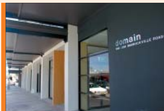
03.44. Solid awnings provide shade as well as rain protection and protect window displays from harsh light and heat.
