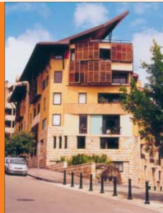
03.56. The feature roof line of this building gives the building a strong identity.
