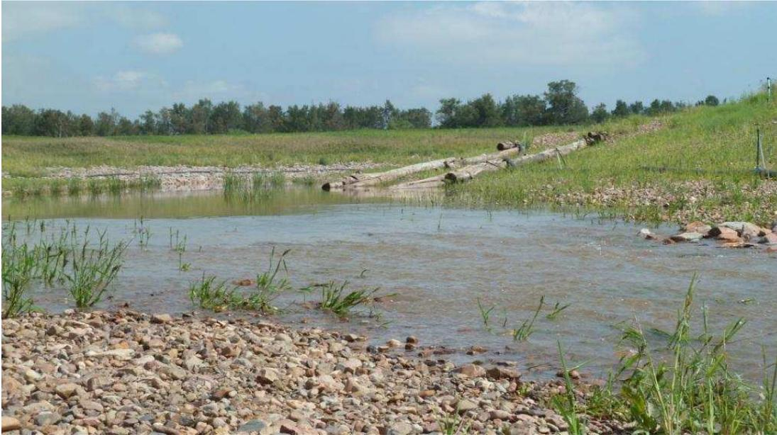
**Further downstream at Bowman’s Creek Eastern Diversion, showing log structures and vegetation planted within the new stream.**
