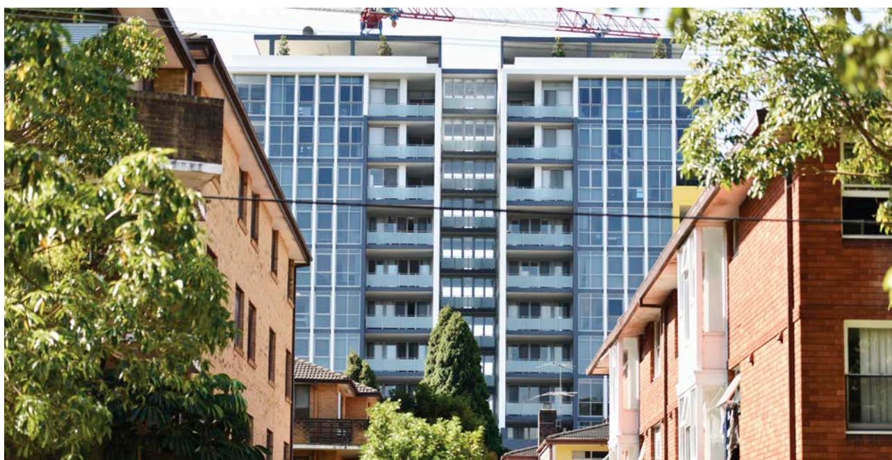
Figure 3. Apartment construction in Strathfield in Sydney’s Inner West
