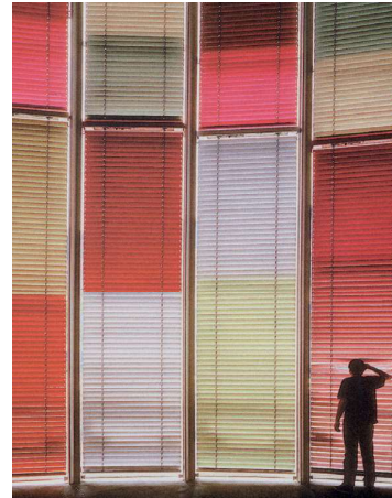
Solar blinds between double glazing reduce heat loads while providing daylight and views.
