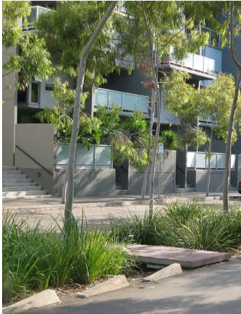
Bio-remediation swales located underneath the street medians filter and redirect the stormwater back into the system for irrigation and various other uses.
