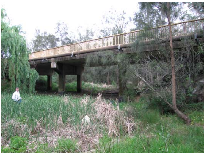
Plate 5 - Bringelly Road Bridge Looking d/s
