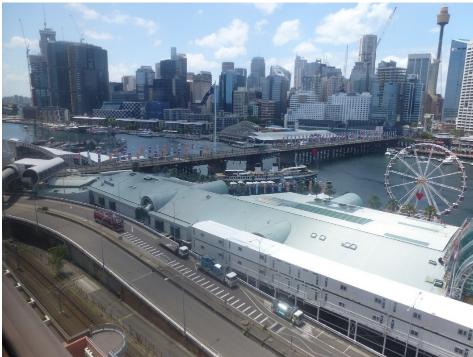
Figure 17 – Harbourside western façade and relationship to Pyrmont Bridge viewed from the west (April 2016) Source: JBA
