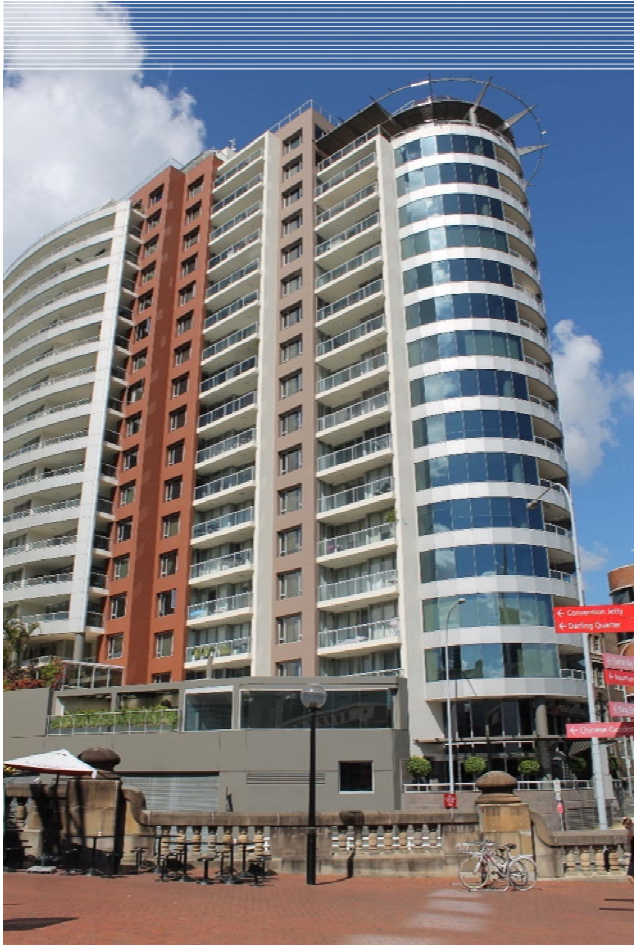
Figure 30 – 50 Murray Street Apartments (November 2016) Source: JBA
