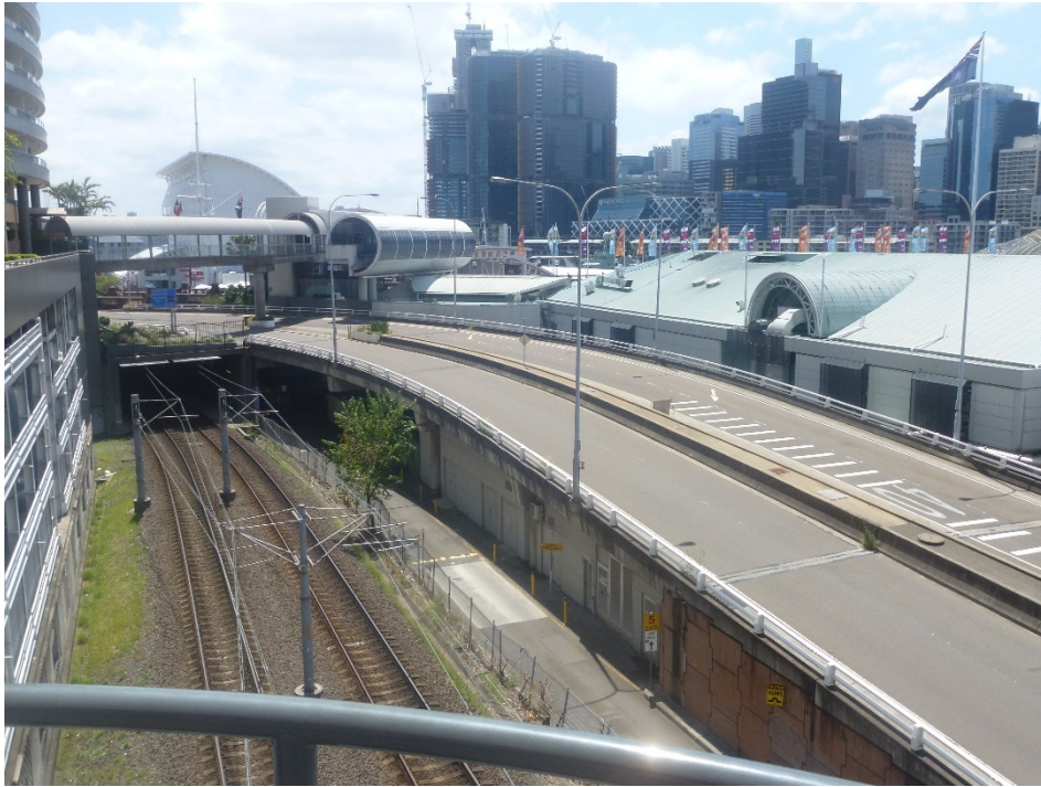
Figure 16 – Northern pedestrian bridge, viewed from the west of the site (April 2016) Source: JBA
