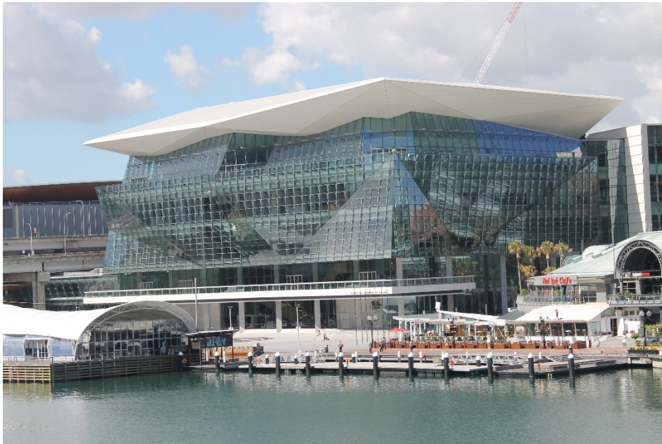
Figure 27 – International Convention Centre (November 2016) Source: JBA
