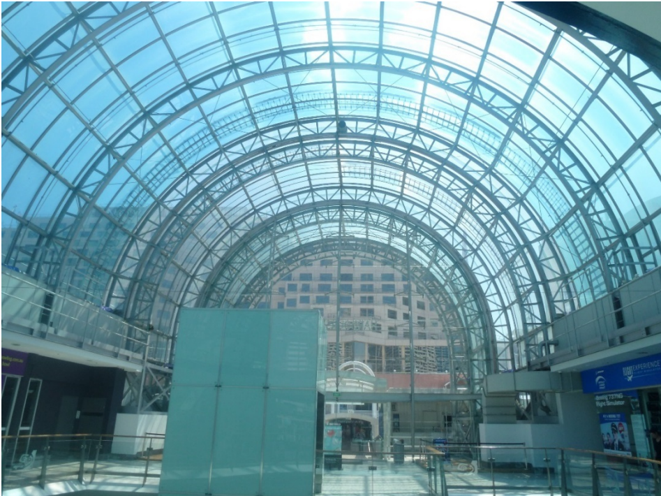
Figure 12 – Internal view of Harbourside (April 2016) Source: JBA
