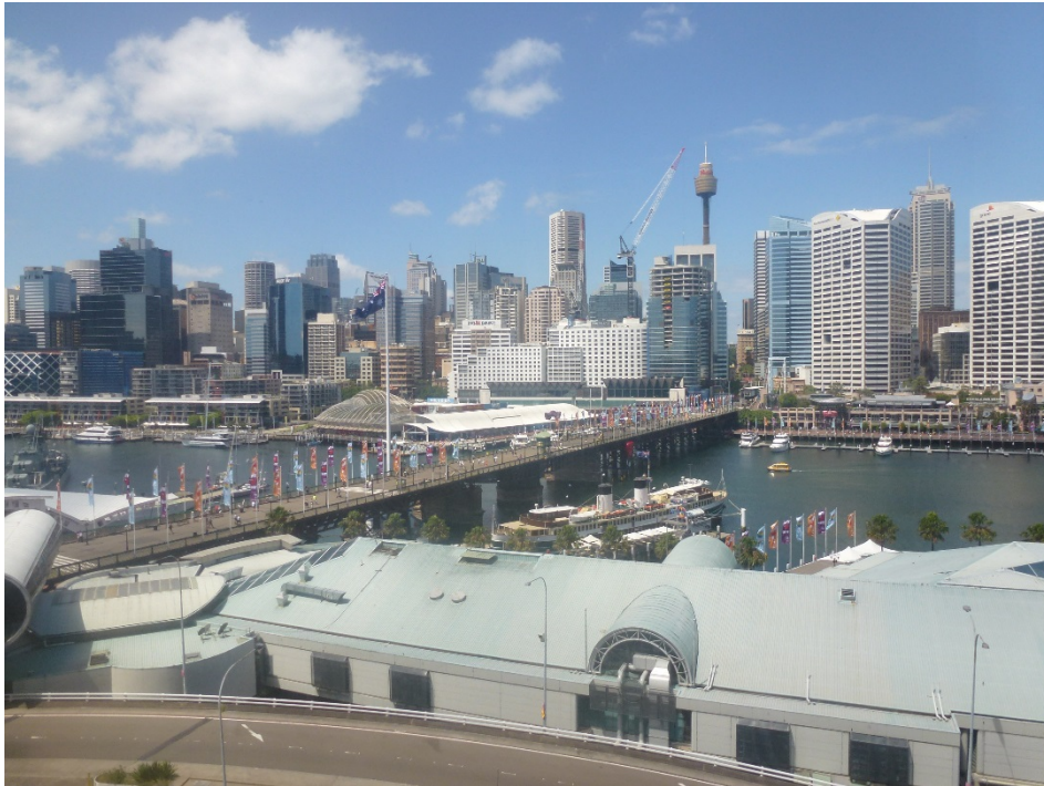
Figure 23 – Pyrmont Bridge viewed from the west (April 2016) Source: JBA
