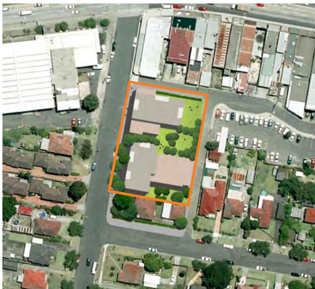
Figure 1C.1 Individual site: this development comprises two apartment buildings with a shared communal open space and mediates between low density housing and a local centre to the north
