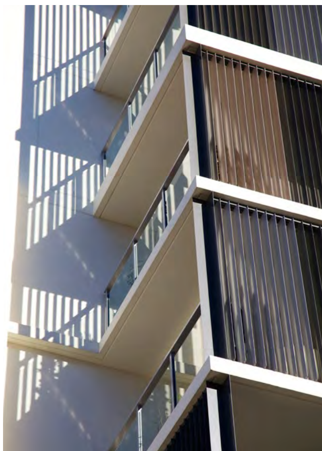
Figure 4A.7 Vertical louvers are an effective sun management technique for east and west-facing windows and balconies
