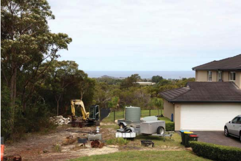
Area 5 Waratah Street view south east
