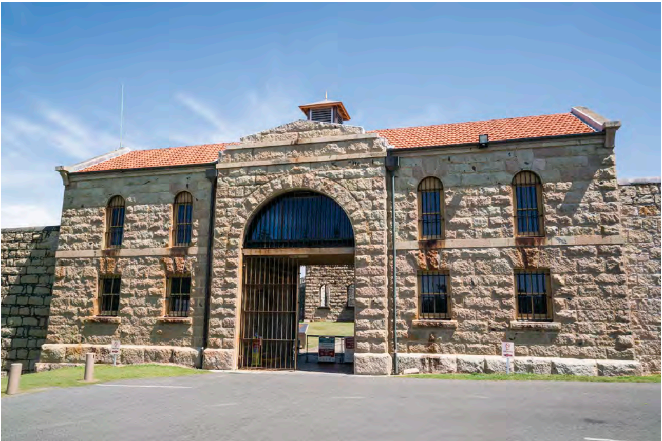
Trial Bay Gaol. South West Rocks, NSW
