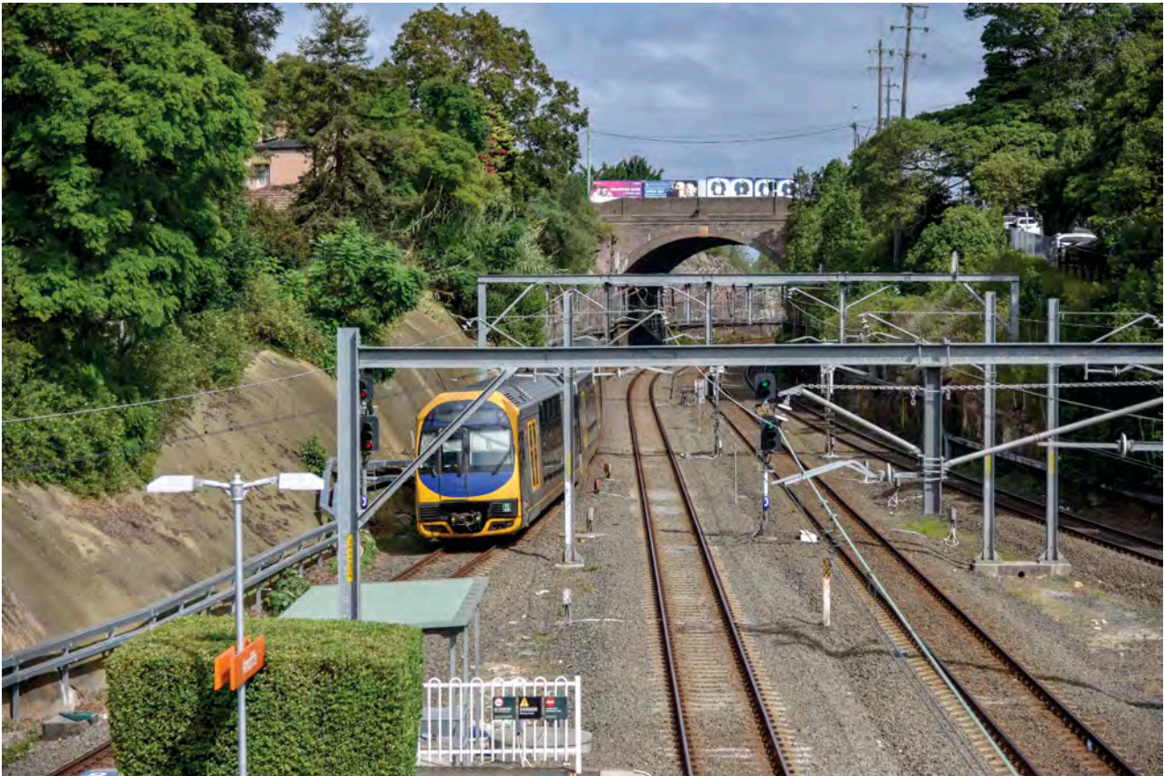
Arncliffe Train Station, Arncliffe, NSW
