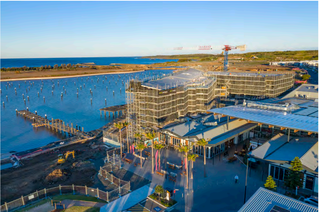
Construction at Shellharbour Marina, NSW
