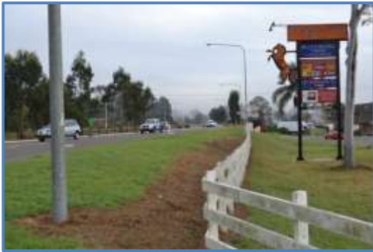
Figure 44 Windsor Road, looking north from Boundary Road.
