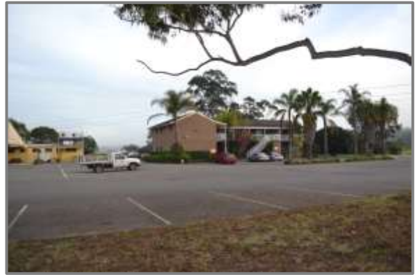
Figure 27 The motel building to the rear of the Vineyard Hotel.
