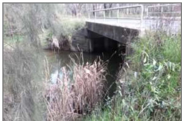
Figure 37 The Chapman Road bridge over Killarney Chain of Ponds.
