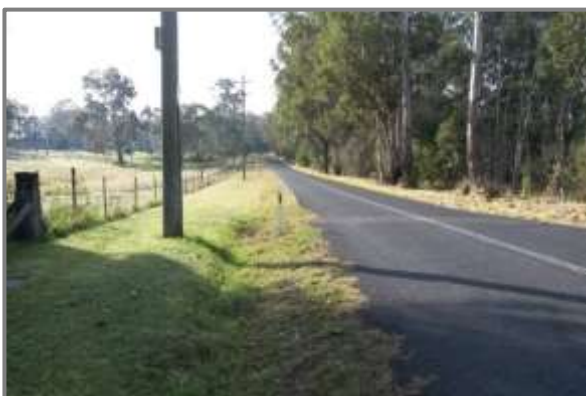
Figure 36 View along Menin Road from Commercial Road.
