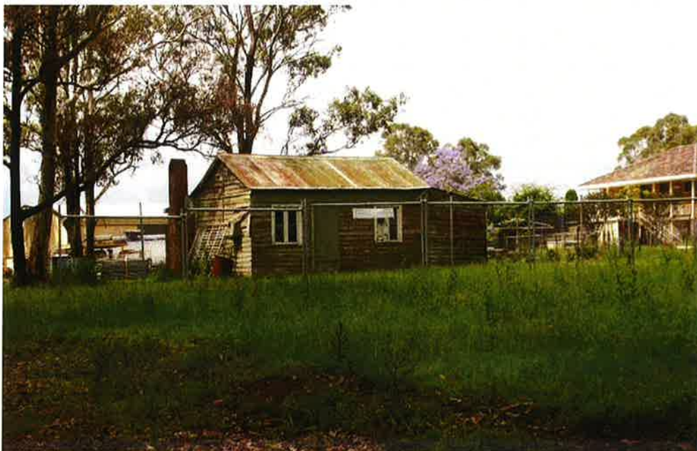
Figure 5.195 The house at 15 Seventeenth Avenue.
