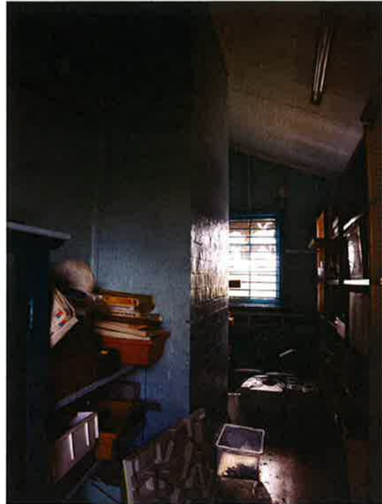
Figure 5.106 Interior partition and rear of brick chimney.
