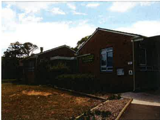
Figure 5.117 Building A, Administration.
