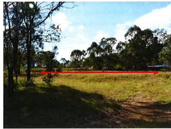
Figure 5.177 Section of embankment along east side of historic road reserve, west of the Upper Canal.
