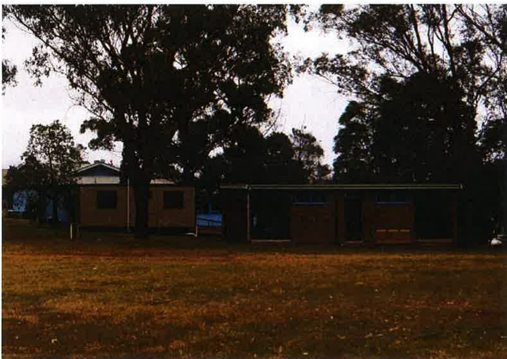
Figure 5.120 Building P (left) and Building G; view from the north.
