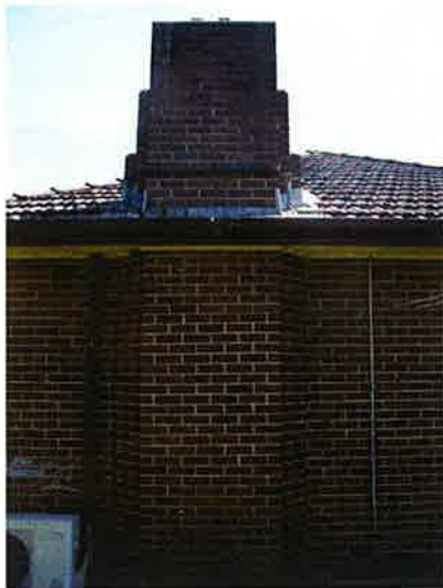
Figure 5.145 Detail of brick chimney, south side of house.
