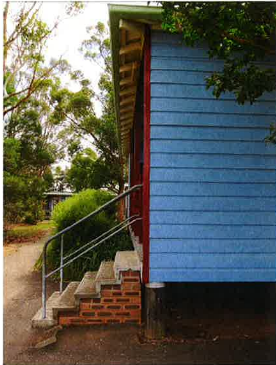
Figure 5.105 Brick stairs with concrete capping, metal safety rails and timber piers.
