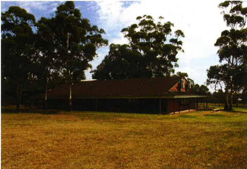
Figure 5.119 Building E, Library.
