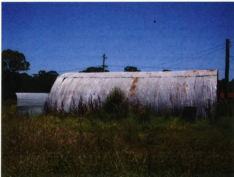
Figure 5.169 The west elevation of the Nissen hut on the corner of Seventh and Edmondson Avenues.
