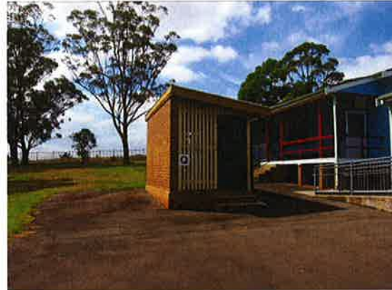
Figure 5.114 Ablution shed (Building Q).
