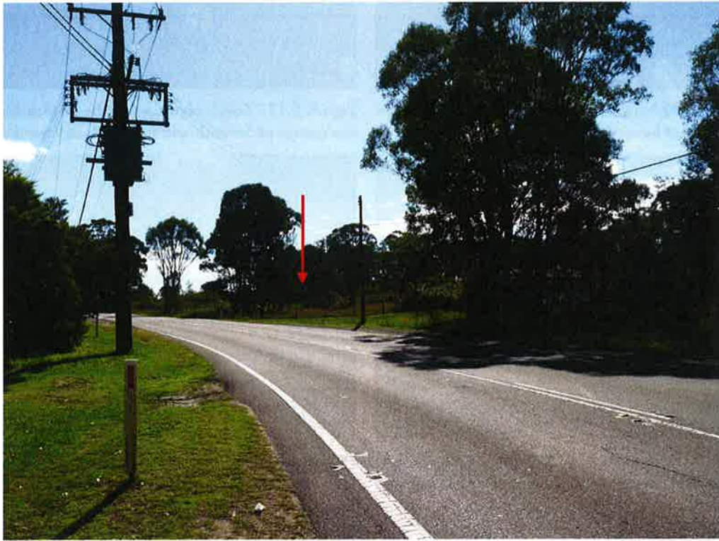
Figure 5.174 A prominent bend in the present Cowpasture Road represents the point at which the road was realigned along the west side of the Upper Canal, following its construction in 1886-1888. A shallow depression along the disused road reserve indicates the original alignment (red arrow.)
