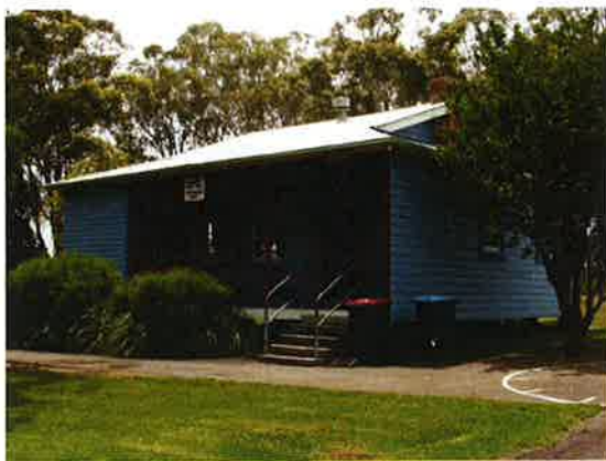
Figure 5.103 Original Raby Public School building, 2011; view from the west
