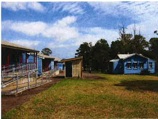
Figure 5.97 From left: group of weatherboard school buildings, ablation shed (Building Q), and original Raby Public School building (Building H); view from the southeast.
