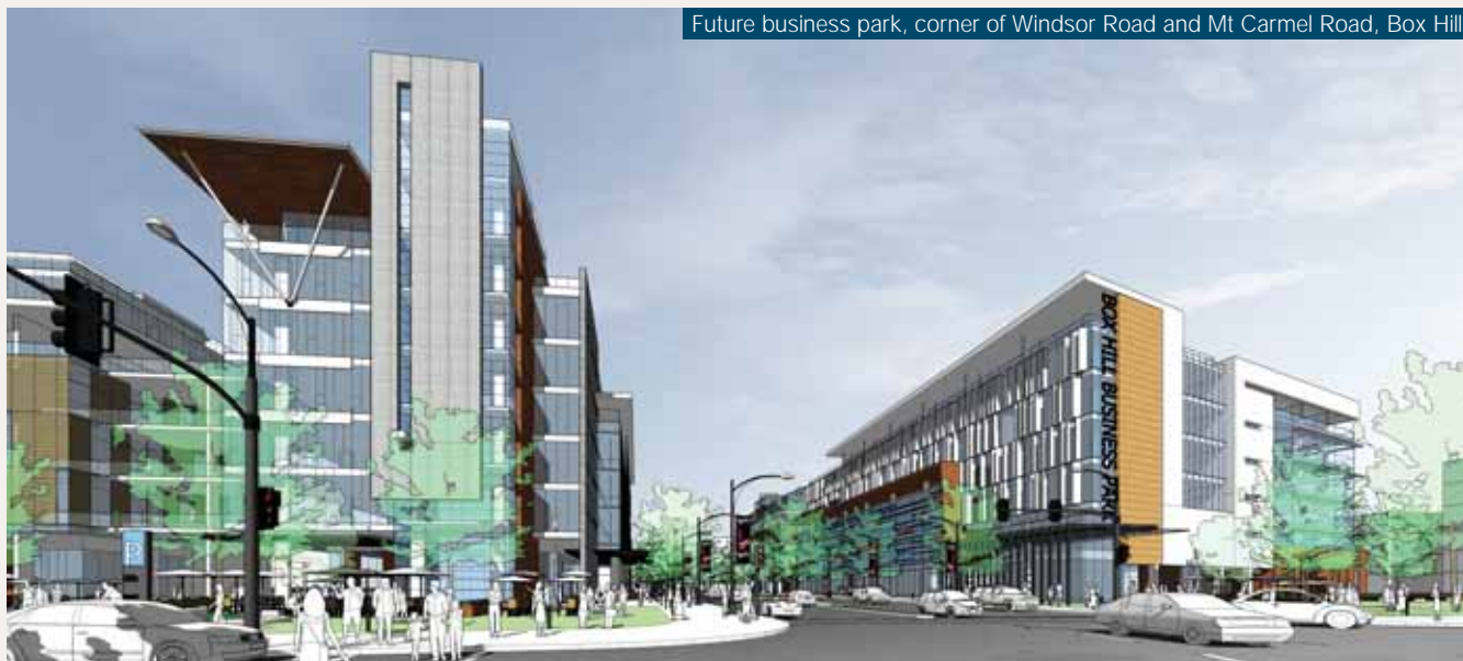
Future business park, corner of Windsor Road and Mt Carmel Road, Box Hill
