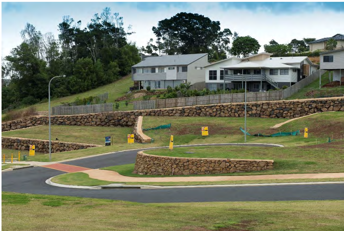
New residential area at Cumbalum in Ballina local government area
