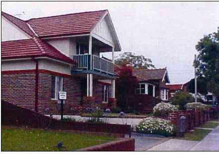
New development can blend into an existing streetscape by using similar proportions, front setbacks and roof forms to adjacent development.
