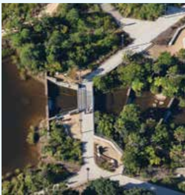
Sydney Park Water Reuse project by Turf Design & Environmental Partnership. Source: Ethan Rohloff Photography.
