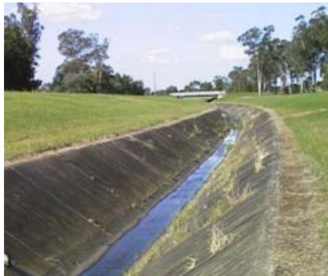
Figure 35: Clear Paddock Creek stormwater drain before works. Source: E2 Design Lab
