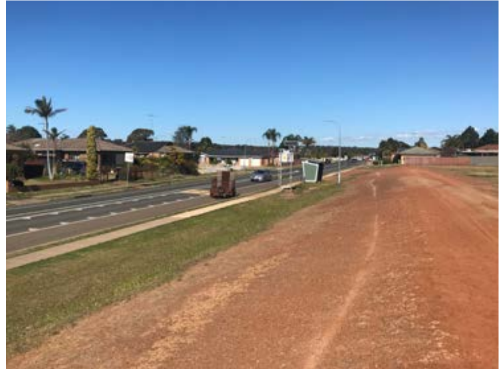
Figure 27: Photograph from the top of existing Haydon Park fill embankment
