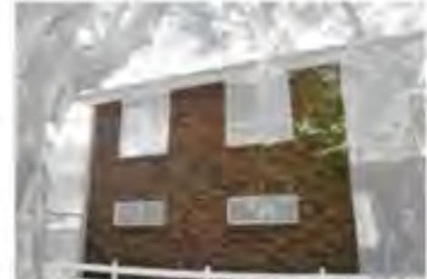
Demolished dwelling bricks recycled into new perimeter walls
