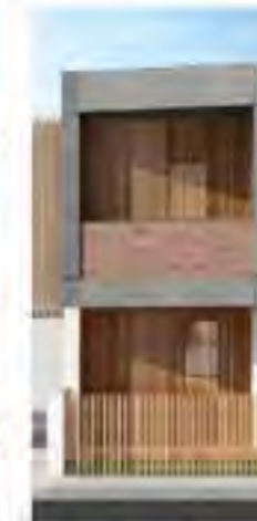
TIMBER SCREENS FOR NOISE/SUN CONTROL
