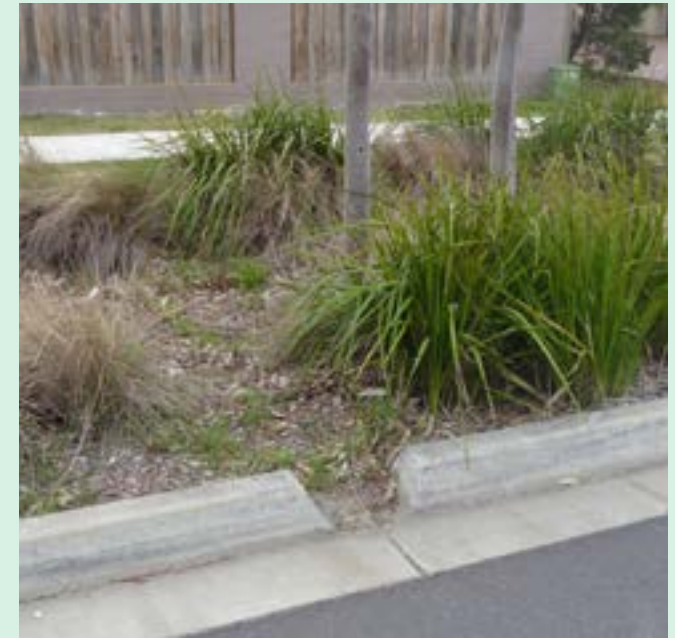
Figure 51: Inlet controlled outlet
