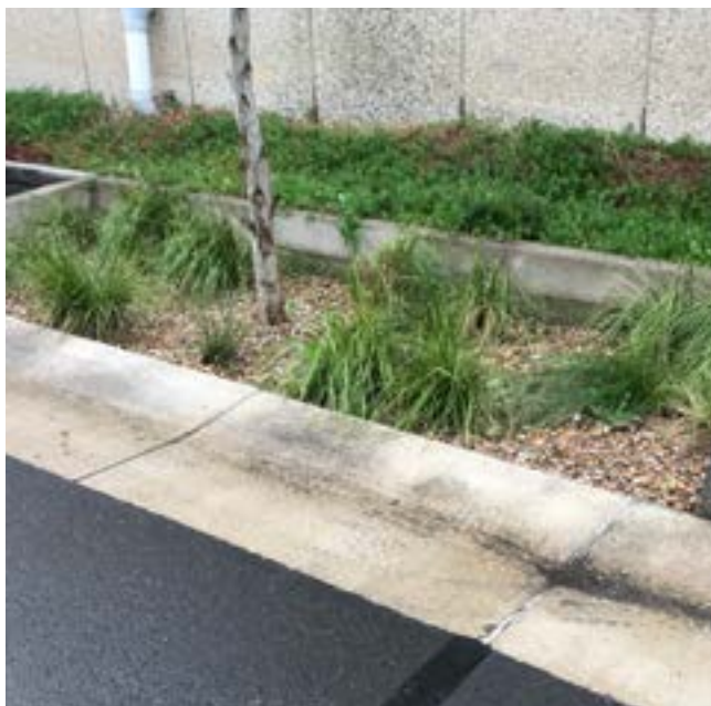
Figure 62: Tree planting dropped below kerb
