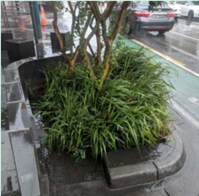
Figure 49: Kerb overflow. Source: E2 Design Lab
