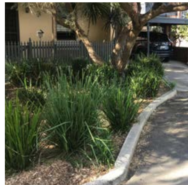
Figure 63: Concrete upstand kerb provides separation of road from pedestrians
