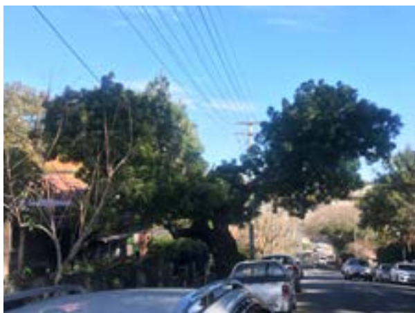
Figure 14: Tree pruned around overhead powerline.
