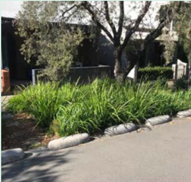
Figure 21: Passive irrigation from stormwater runoff
