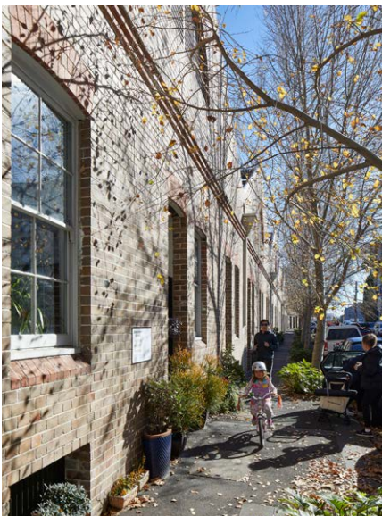
Figure 8. Retention of heritage facade at The Gantry by Bates Smart. Image: Martin Mischkulnig
