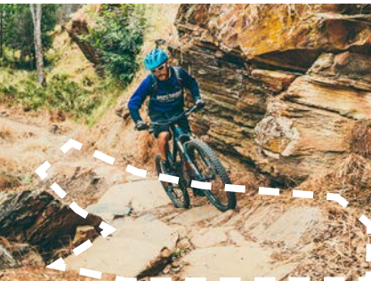
Trail armoring. Armoring is a method of using large rocks to pave a trail and prevent erosion.
