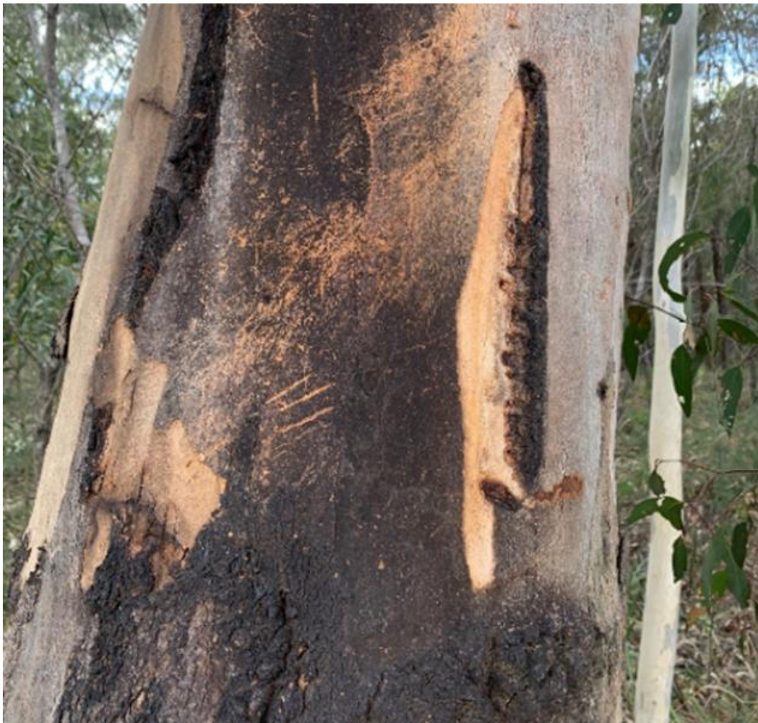
Figure 3. Koala claw marks sighted by the CPCP team at Kings Falls Bridge
