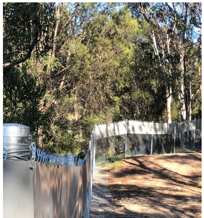
Figure 10: Koala-exclusion fencing adjacent to a fire trail in Appin
