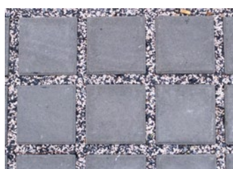
Concrete unit paving and gravel joints
