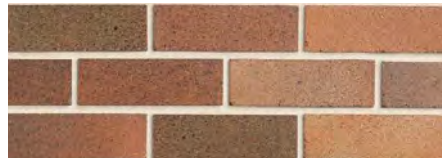
WF2 - Brick walls Face brick - lighter top Colour-matched mortar
