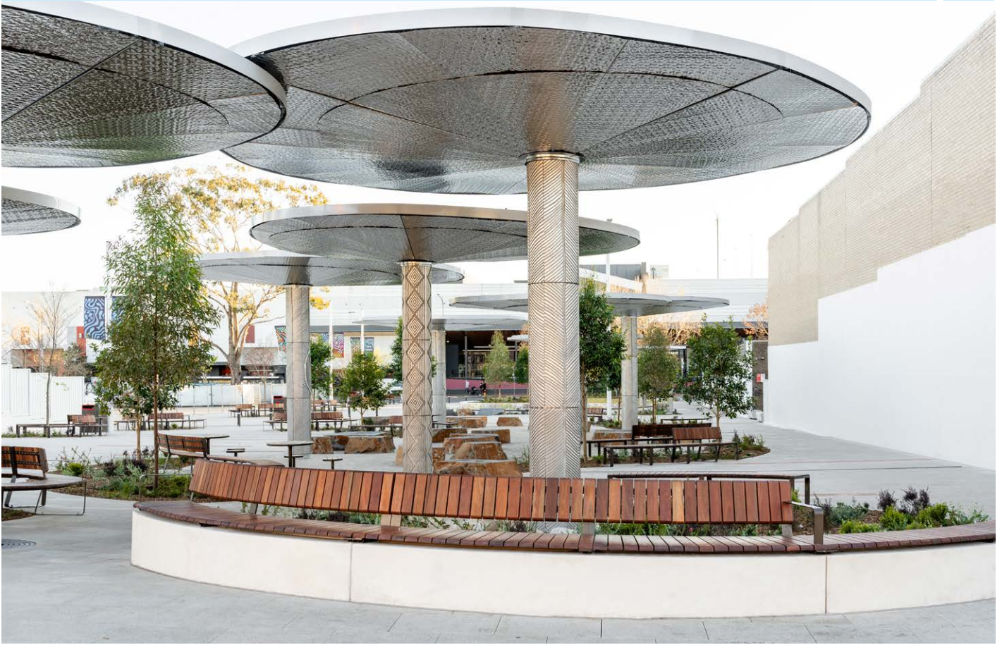
Image 3: Merrylands Civic Square. Completed in 2023 and funded by the NSW Public Spaces Legacy program. Credit: Cumberland Council.
