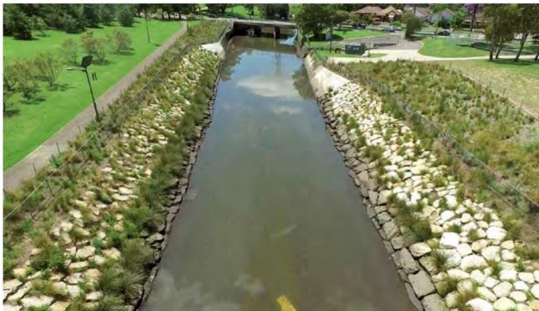
Figure 5-3: Potential lowered bank profiles
